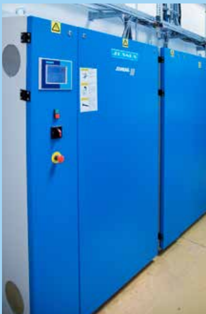
Control centre of the Jenrail 2000 Automatic system with Jentrol HMI PLC and touch screen.
