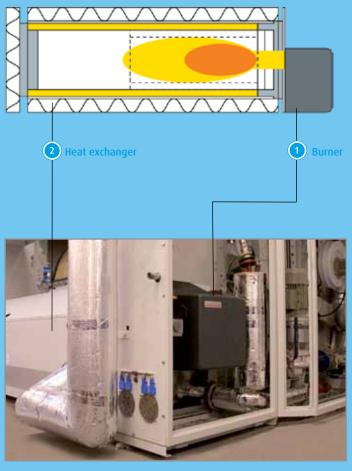
Integrated gas-fired burner and heat exchanger
